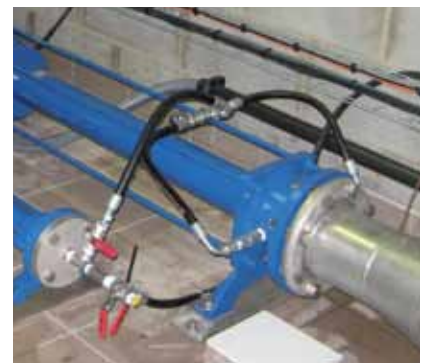
Polymer lubrication incorporated in GBB in transfer of dewatered sludge with or without lime treatment.
