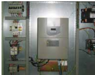
Level control in lime treatment applications.
