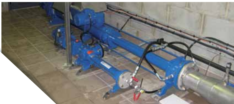
Polymer lubrication incorporated in GBB in transfer of dewatered sludge with or without lime treatment.
