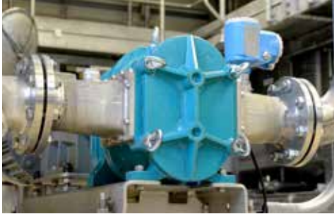
BLUEline pump for conveying cleaning agent
